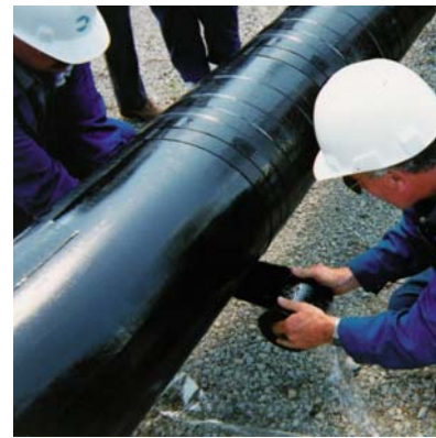
Application of Denso 60 Tape.
