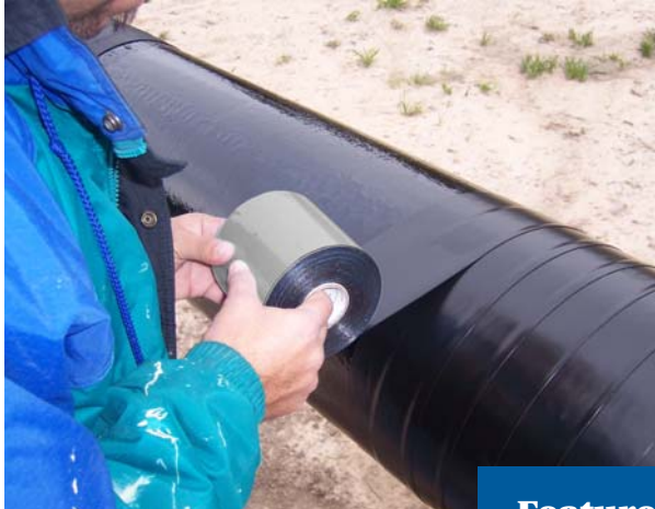
Application of Denso Butyl 35 Tape.
